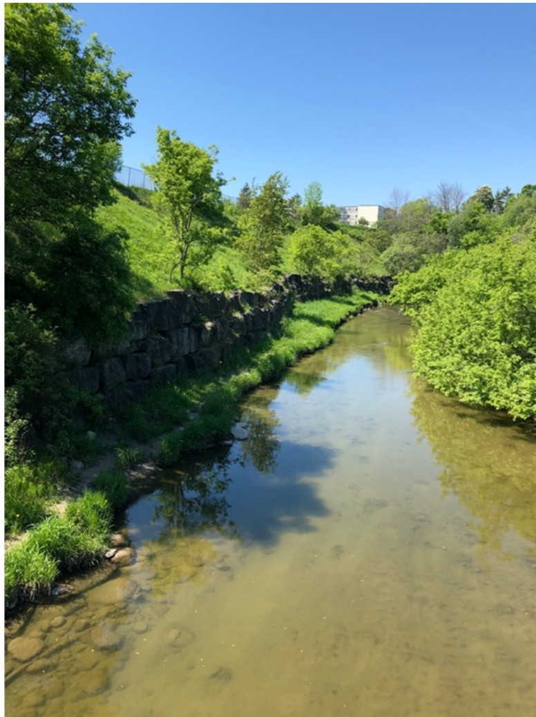
City of Courtenay, BC, project
